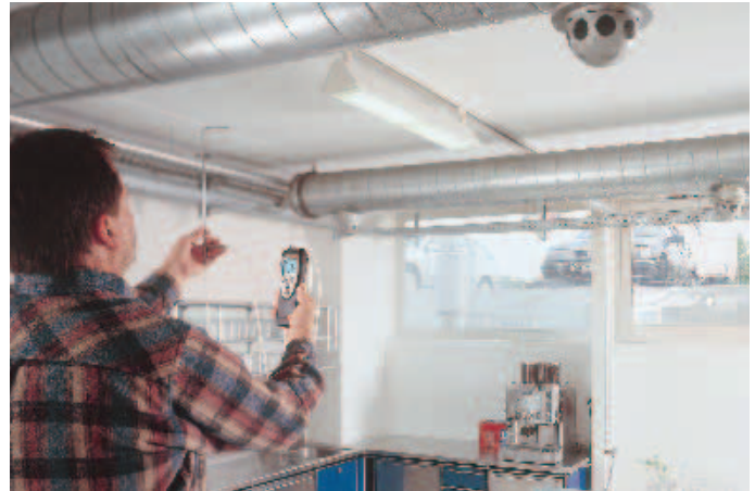
Measuring outlet air
